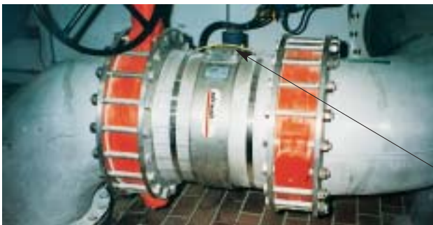
Waste water treatment plant Frankfurt-Sindlingen Electrical conductivity through external cable connector (made on site) STRAUB-FLEX 2LS used as main joint.
